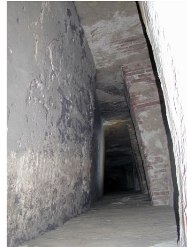
Interior walls of Brunelleschi’s double cupola
